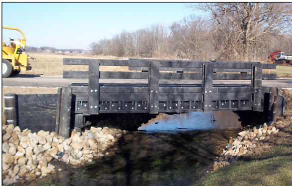
Bridge 174-0.56 over the Onion Ditch
